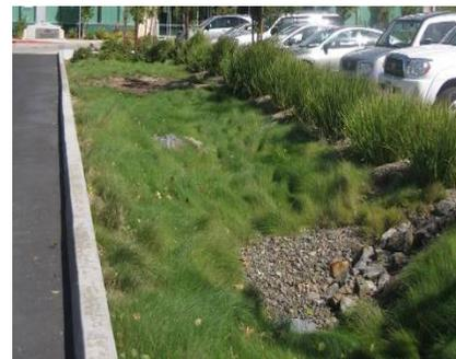
Figure 5-3. On-site storm water capture through landscaped swales.
