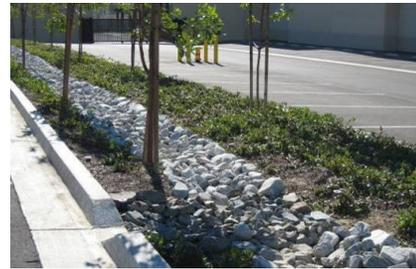
Figure 5-2. On-site storm water capture system.
